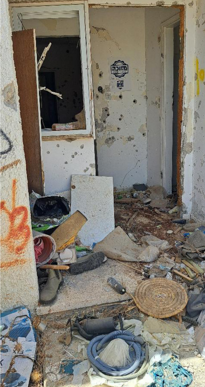
FIG. 1. One of the many destroyed homes of Kfar Aza. Note the shoes in the entryway. Courtesy of Karen Shawn.
